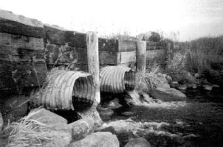
Figure 2. Downstream view of a stream crossing that is a high priority for maintenance because of excessive perch ( > 0.2 m) and high water velocities ( > 0.35 m/s) that present a potential passage problem for Topeka shiners.
